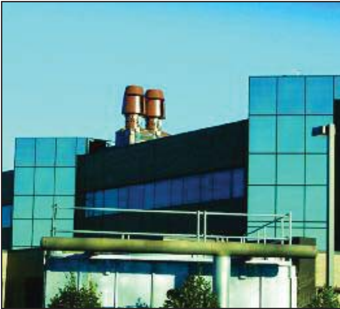
■ Figure 2. Mixed-flow impeller fans have a low profile, typically measuring about 15 ft high.
