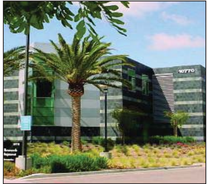
■ Figure 3. There you see it, here you don't. To comply with local ordinances governing roofline aesthetics, the mixed-flow impeller systems are mounted inside the building of this pharmaceutical manufacturer.
